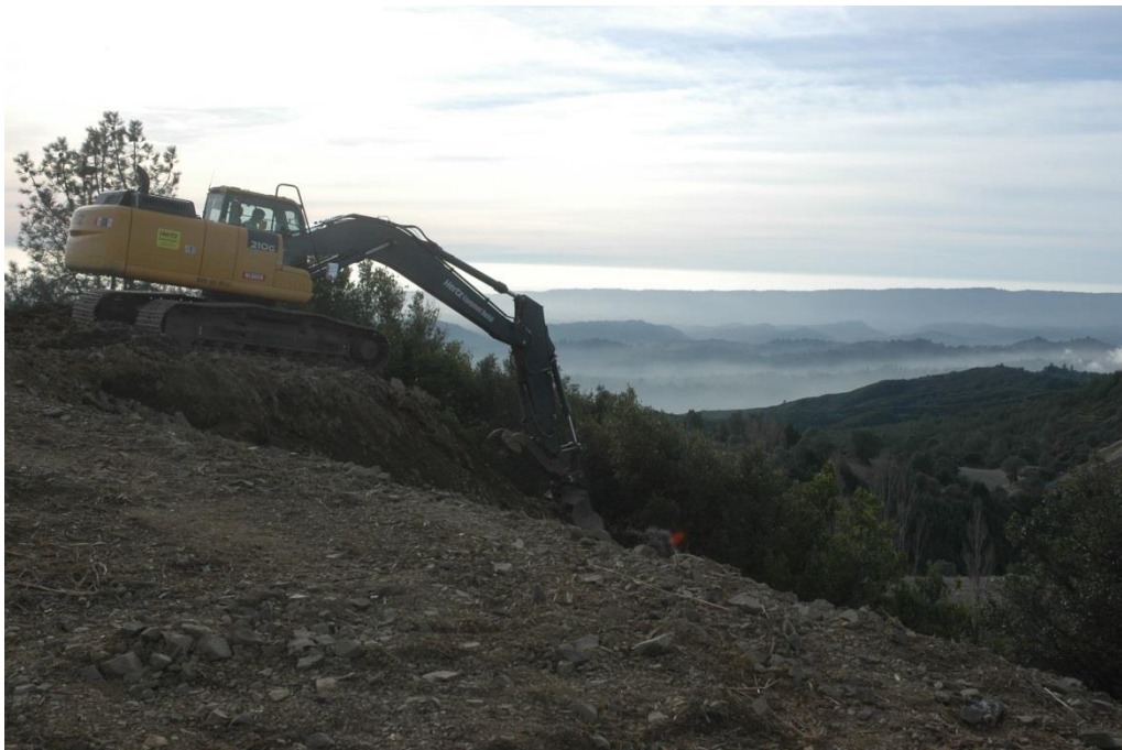
Figure 2. As the vegetated edge of the summit is pulled back, the existing root channels and soil structure is mixed. Existing root channels and drainage pores are destroyed. Mixing of coarse wood materials and care to not re-compact the substrates are the primary treatments to regenerate pore space for root growth and drainage.
