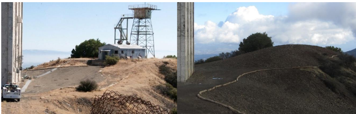
Figure 5: Before and after photos of re-contoured east summit area after rough grading and structure removal. Grading will be refined in 2016-2017.
