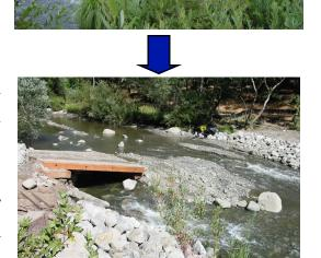
The 2006 removal of Niles Dam allowed fish to once again move freely through this part of the canyon. This 6-ft high dam from the 1880's blocked fish passage at all but the highest flows, and no longer served a useful purpose. Its removal immediately provided migrating fish with an additional 5 miles of high quality
